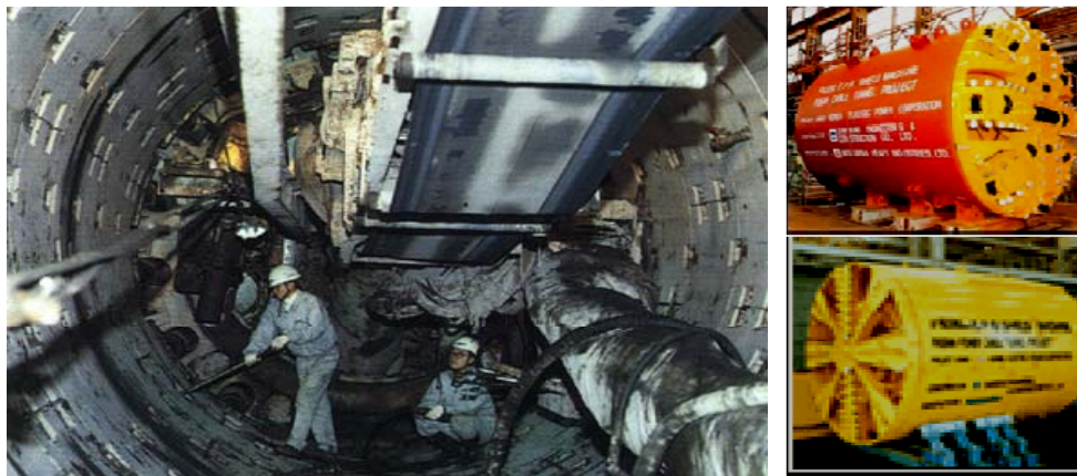
TBM tunnel boring machine
